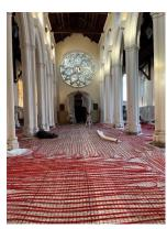
Progress - There has been significant progress over the last few weeks. The underfloor heating engineers have finished laying all the heating pipes and the system has been pressure tested. This week the limecrete is being poured over the floor. This will cure over the Christmas break ready for the York stone slabs to be laid in January. The timing for the laying of the limecrete is critical to allow it to dry over Christmas and we are really pleased that the project is running on schedule.
